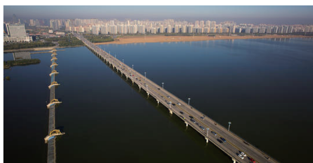
The lifting engineering of Yihe Bridge, Beijing Road, in Linyi, has a total length of 1210.72 meters, a lifting height of 3.1 meters, and a lifting area of 2680 square meters. The lifting engineering of Yihe Bridge in Shangdong province is the lifting and reconstruction engineering of single bridge with the largest synchronous lifting area and longest length in China.
