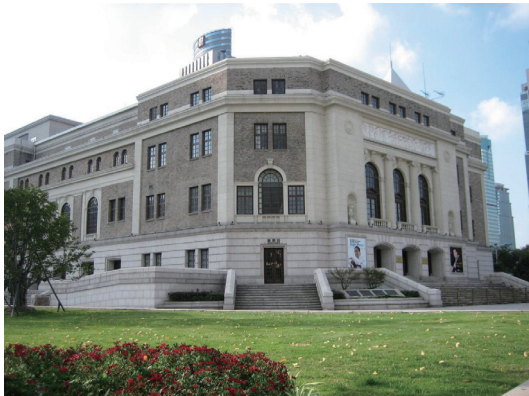
The moving and lifting engineering of Shanghai Concert Hall, covers an area of 1,300 square meters, weighs 5650 tons, has a translation distance of 66.46 meters, and a lifting height of 3.38 meters. The PLC synchronous computer control system in the moving and lifting engineering of Shanghai Concert Hall is applied in the translation and lifting engineering for the first time, creating a milestone in the translation and lifting
