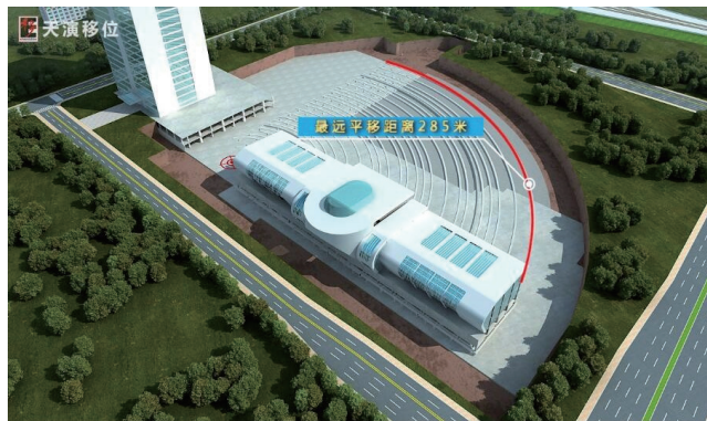
The translation and rotation engineering of Houxi Station main station room in Xiamen, the moving building area are 21764 square meters, the total weight are 32,000 tons, and the longest arc of the building’s rotation and translation are 288.24 meters. The translation and rotation engineering of Houxi Station main station room in Xiamen has won the Guinness World Record of "the longest arc length of the entire building’s rotational movement".
