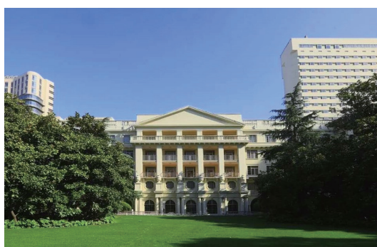
The overall lifting engineering of the South Building of Huadong Hospital in Shanghai, the construction area are 10702 square meters, weighs 25000 tons, and has a lifting height of 1.2 meters. The overall lifting engineering of the South Building of Huadong Hospital in Shanghai is now the largest cultural relic building lifting and seismic isolation reconstruction engineering in the country.
